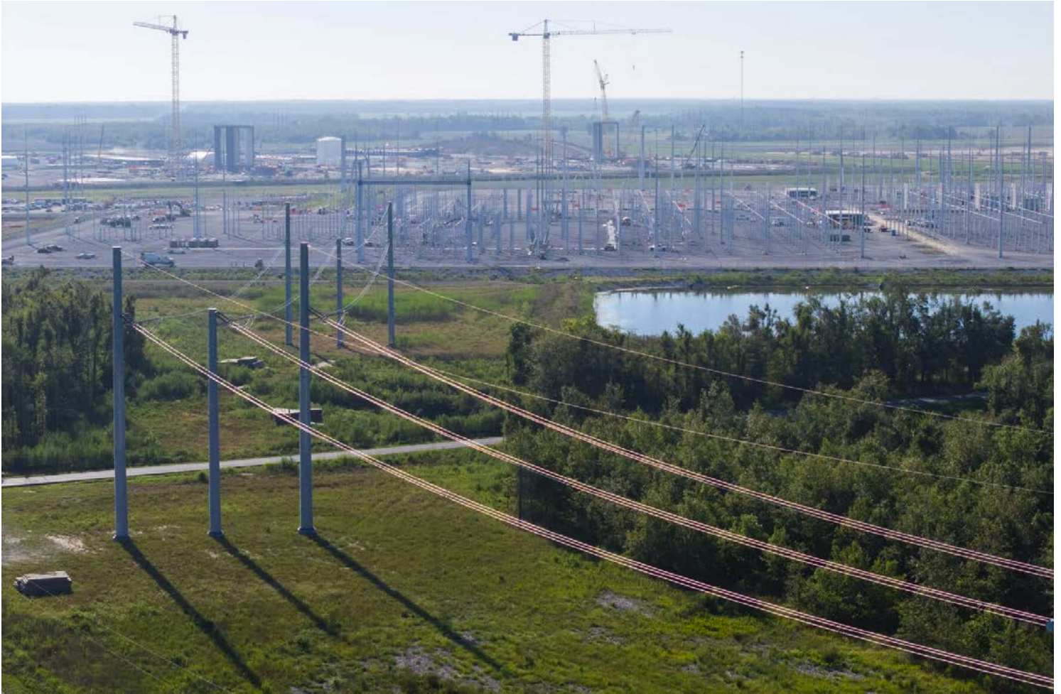
Electrical lines lead to the Meta Hyperion Data Center site in Richland Parish, La., Wednesday, Sept. 2, 2026. (Staff photo by Sophia Germer, The Times-Picayune)
