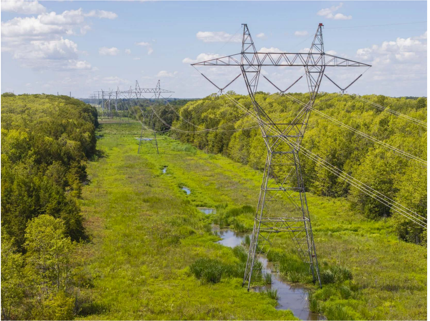
Transmission towers span over Calhoun brake, owned by the Perry family, in Ouachita Parish, La., Tuesday, Sept. 1, 2026. (Staff photo by Sophia Germer, The Times-Picayune)
